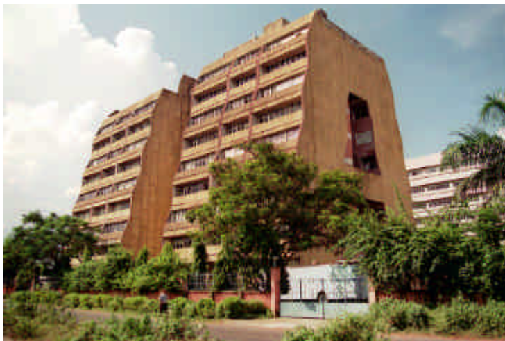
NCSM Headquarters and CRTL facilities at Kolkata
